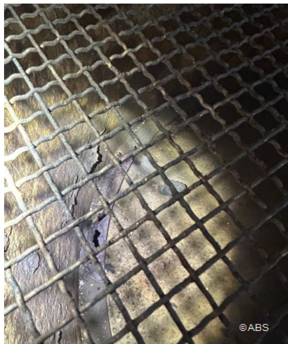
Fire damper flap wasted
